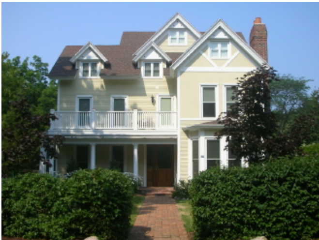
SITE 7 -- DUTCHER-MARK HOUSE | 1889 148 Union Street, Douglas
